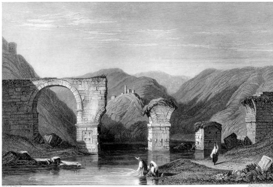
BRIDGE OF AUGUSTUS, AT NARNI.
